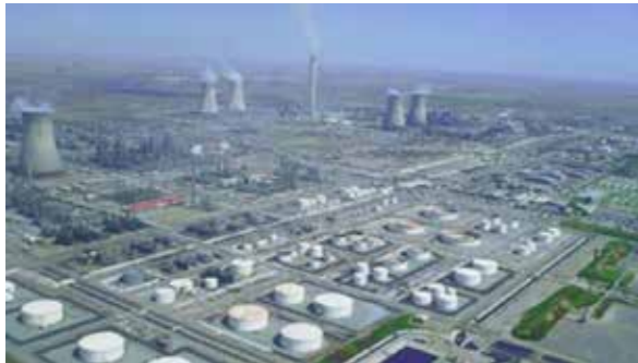
Coal To Liquids plant, Secunda, G. Afrika
