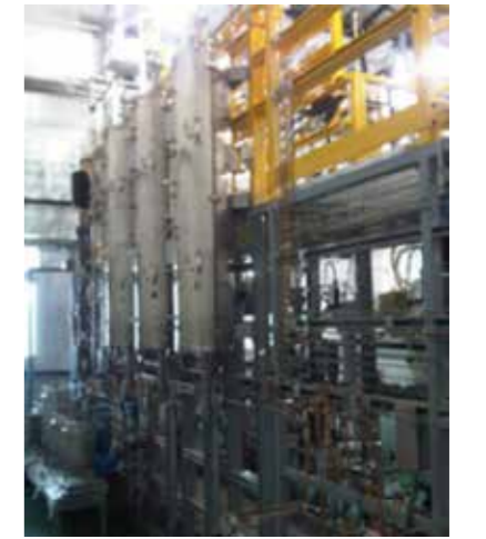
Whole Fraction Tar Upgrading Pilot Plant at National Institute of Clean and Low Carbon Energy (NICE), China
